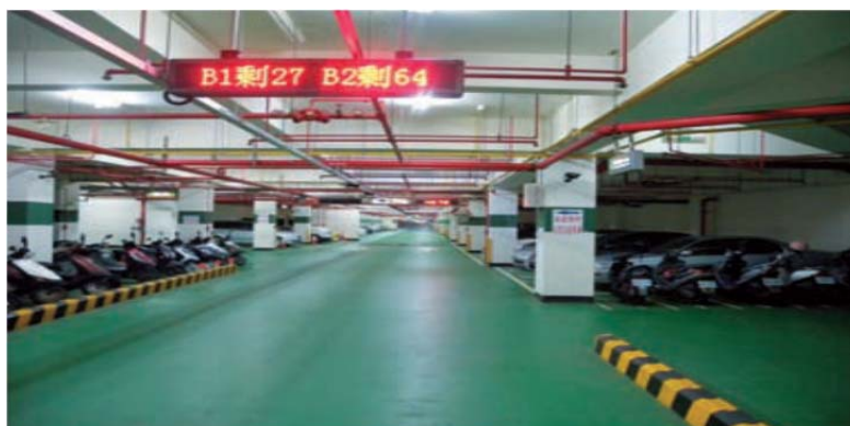
Figure 3: Smart signage system displays occupancy and allows drivers to look for available parking spaces.
