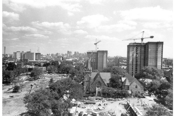
Student residential towers under construction in the late 1960s. Image provided by the University of Pennsylvania.
