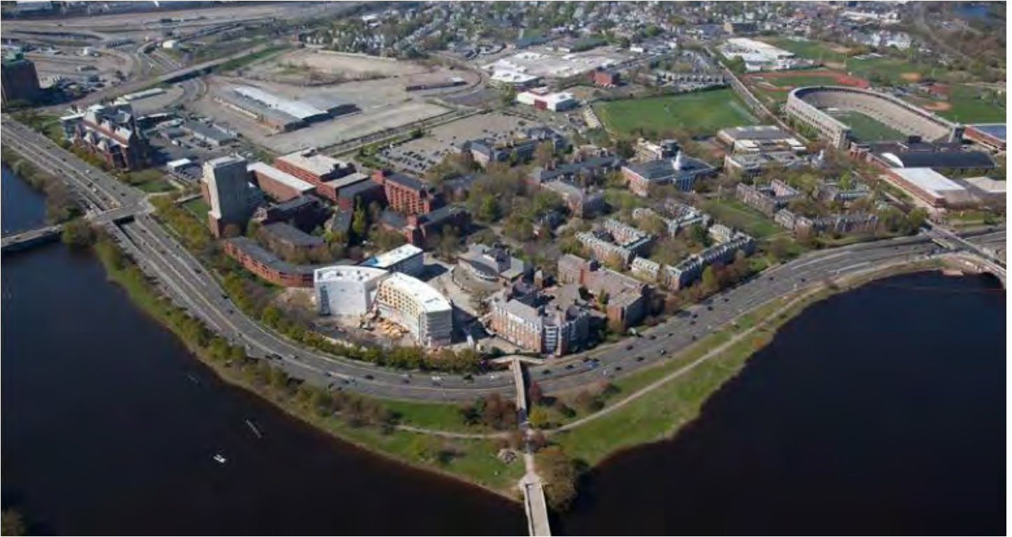
Existing conditions including the Allston Campus and Weeks Pedestrian Bridge. Photo by Mark Flannery.
