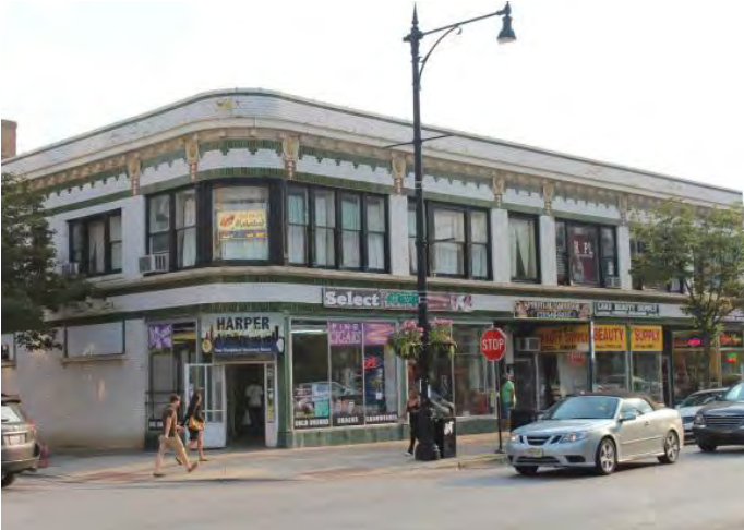
Pre-revitalization conditions on 53rd Street. Photo provided by University of Chicago.
