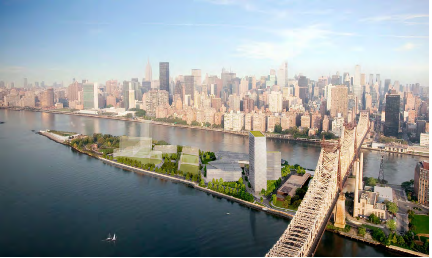
A rendering of the Cornell NYC Tech campus at full build-out. Image provided by Cornell Tech.
