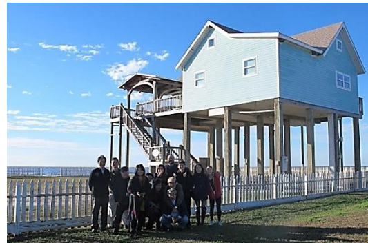
Many residents of Bolivar Peninsula, a coastal community minutes from Galveston Island, have rebuilt their homes to withstand the next hurricane and storm surge.
