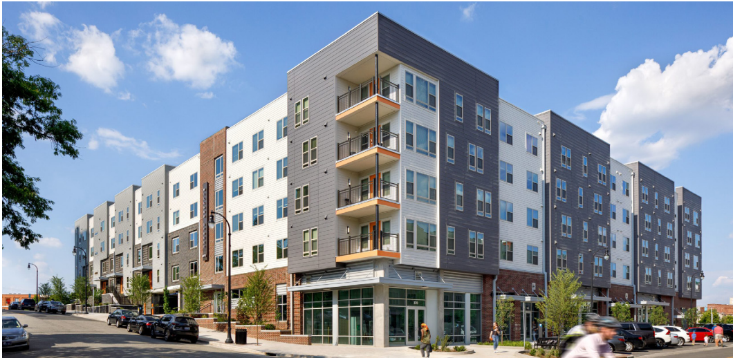
Figure 4 Willard Street Apartments (DHIC n.d.)
