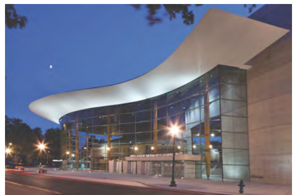
Above, historic facilities. Below, Arena Stage exterior after renovation.
