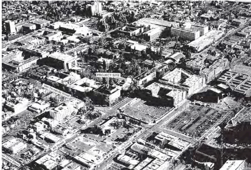
Site before demolition of Wahlquist Library. Source: King Library Archives.
