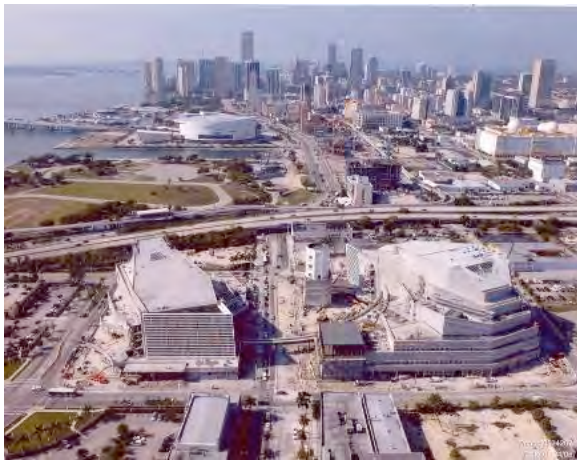
Construction of the Arsht Center with downtown Miami beyond.
