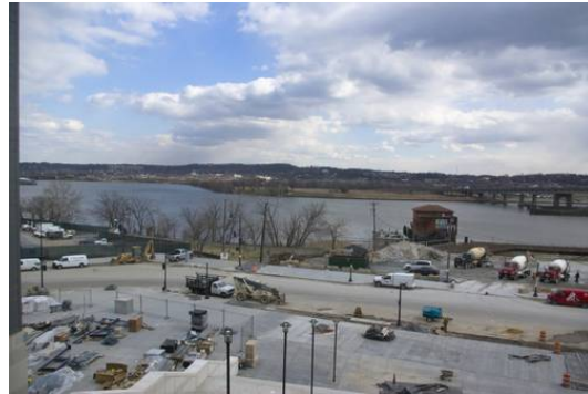
Aerial showing ballpark in center left, above. View from ballpark toward Anacostia River, below.
