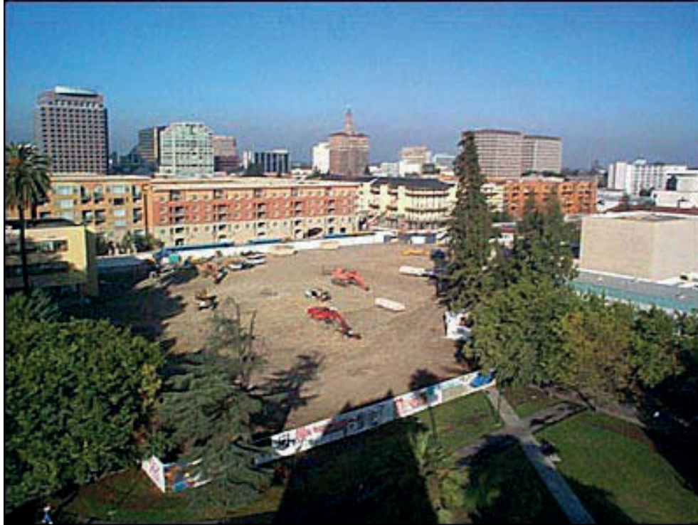
Library site after Walquist Building demolition.
