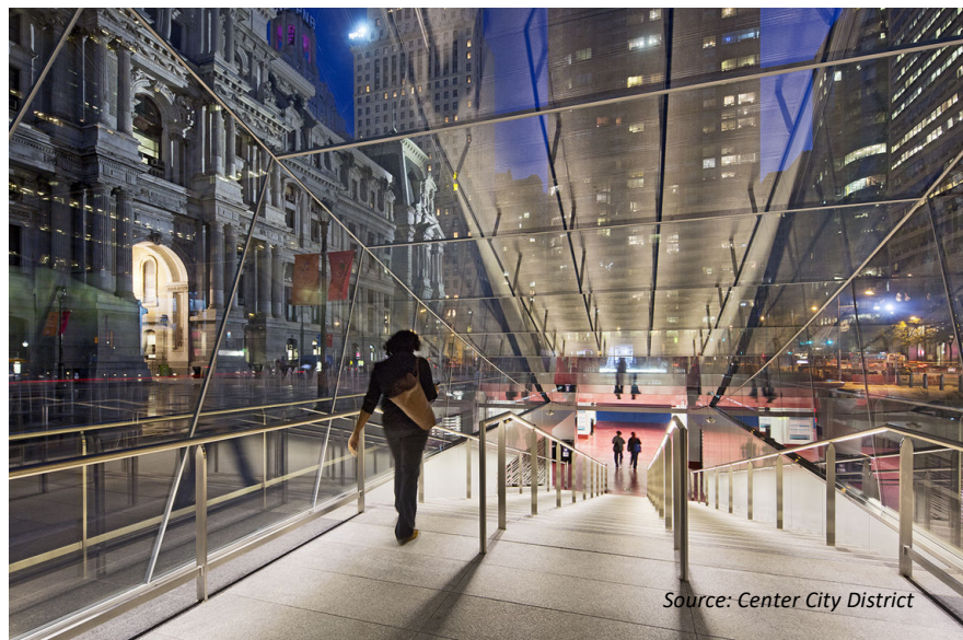
Figure 9 New subway entrances in Dilworth Park
