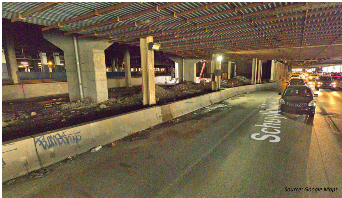
Figure 18. I-76/ Schuylkill Expressway under 30 th Street Station and the Porch
