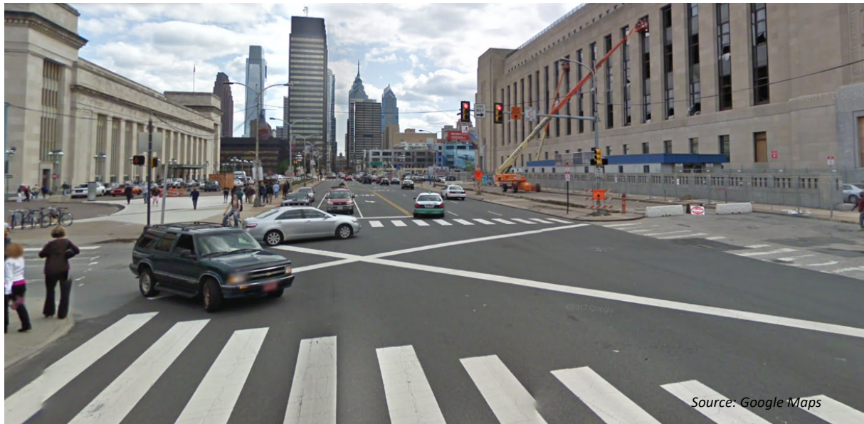
Figure 15. Market Street, September 2009. Facing east, Station on the left; Post Office on the right; 10 drive lanes, 3 parking rows, poor sidewalks and no trees.
