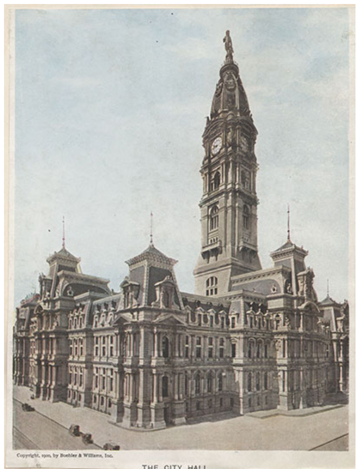
Figure 6 Newly Constructed City Hall in 1892
