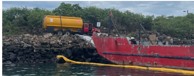
Photograph from Site Visit: Fuel Transfer Process in San Cristóbal
